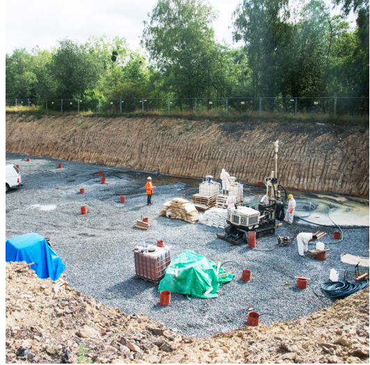
Direct push injection of the persulfate/calcium peroxide mixture
