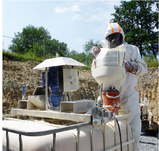
Preparation of the persulfate/calcium peroxide suspension
